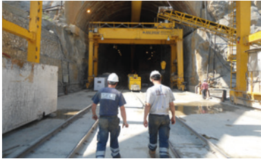
"KISHANGANGA" HYDROELECTRIC PROJECT ASIA
